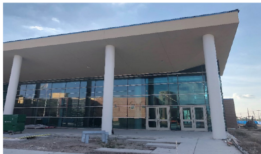
Eastern view of new addition
